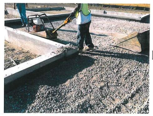
Placing Base for floor slabs
