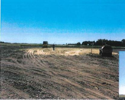
Placing Embankment and working subgrade.
